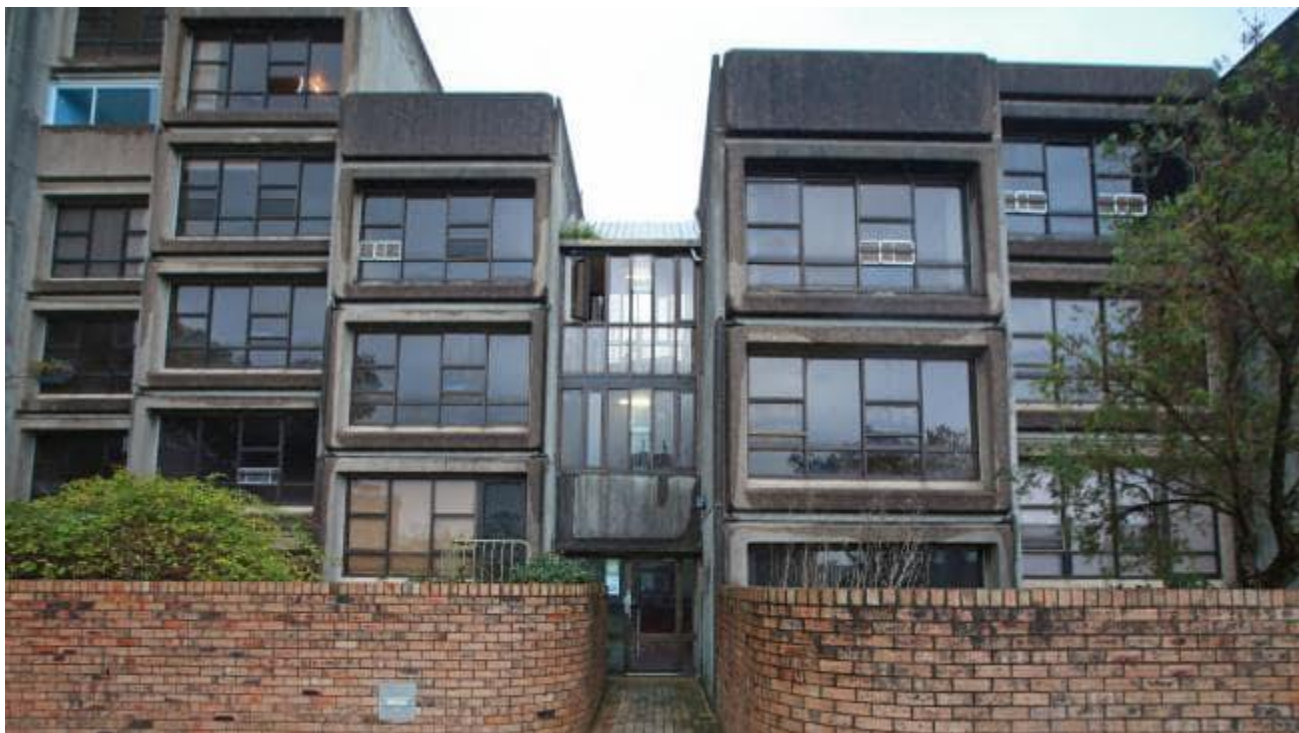
Sirius Building at The Rocks was built in 1979 to accommodate social housing tenants. Picture: Cameron Richardson
